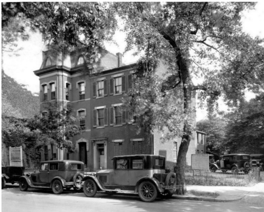
The future site of the second church building at 1906 H Street, NW
